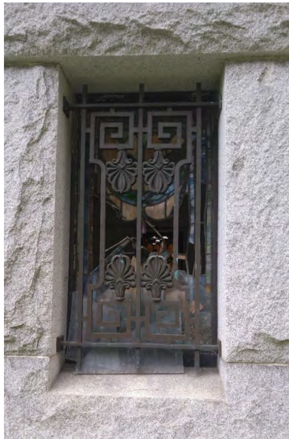
Figure 26. Shattered window and twisted lead from frost action
