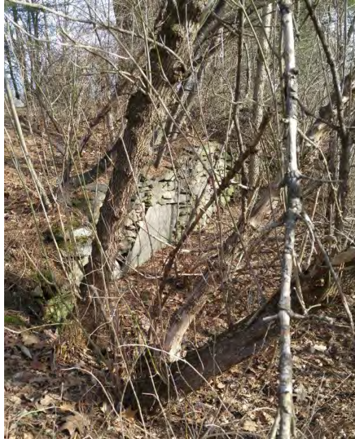
Figure 23. Stone retaining wall
