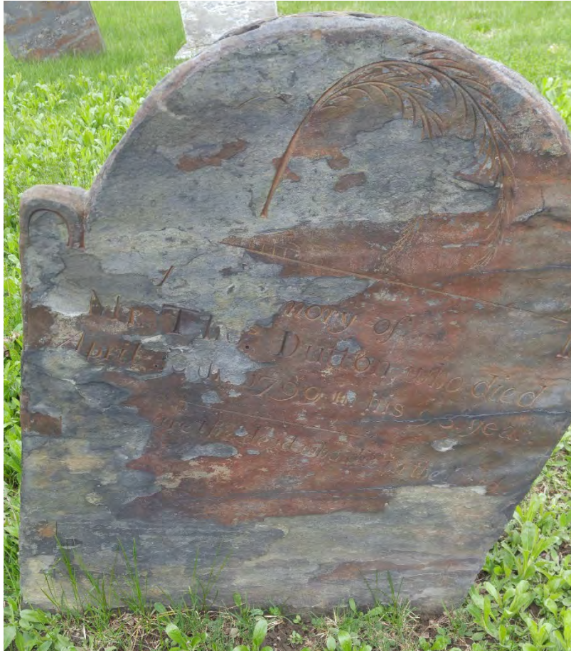
Figure 20. Partially delaminated stone (1799) possibly from Bartlett's quarry
